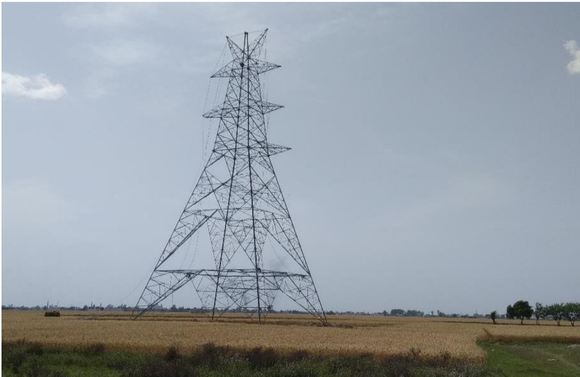
Location 35/0 – Tower erection progress
