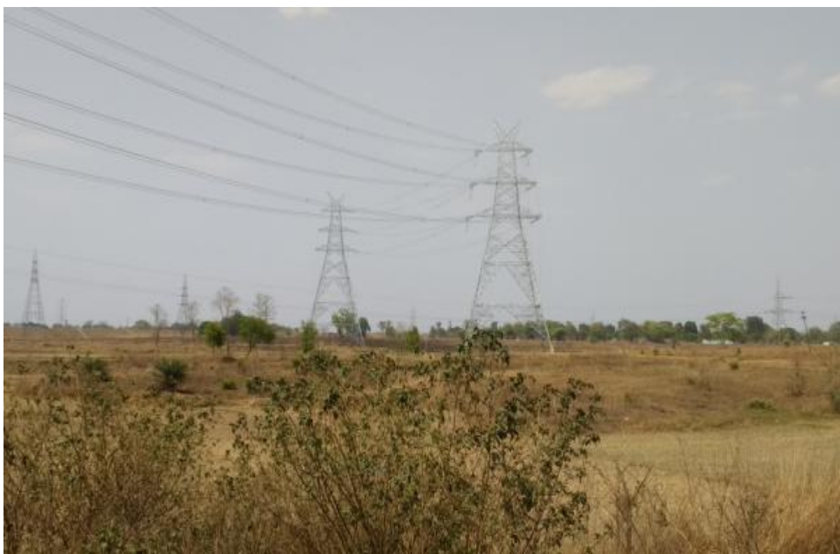
Stretch 30/0(DD+18) to 35/0 (DC+0) – stringing complete
