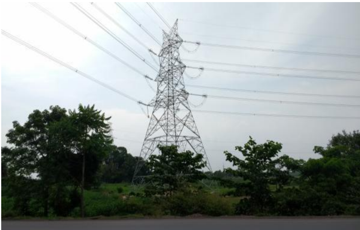
Location 32/0 – Road crossing, Erection and stringing complete
