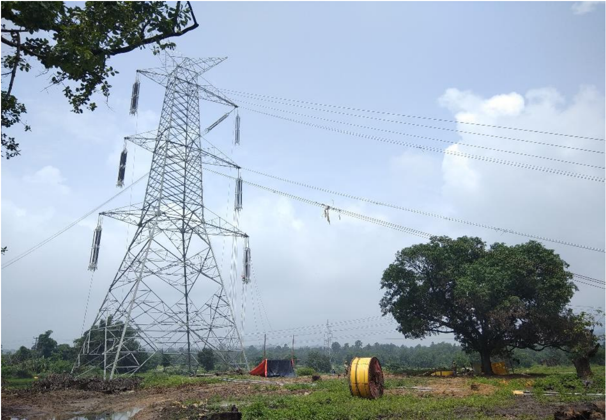
Location 115/0 – Stringing works are in progress
