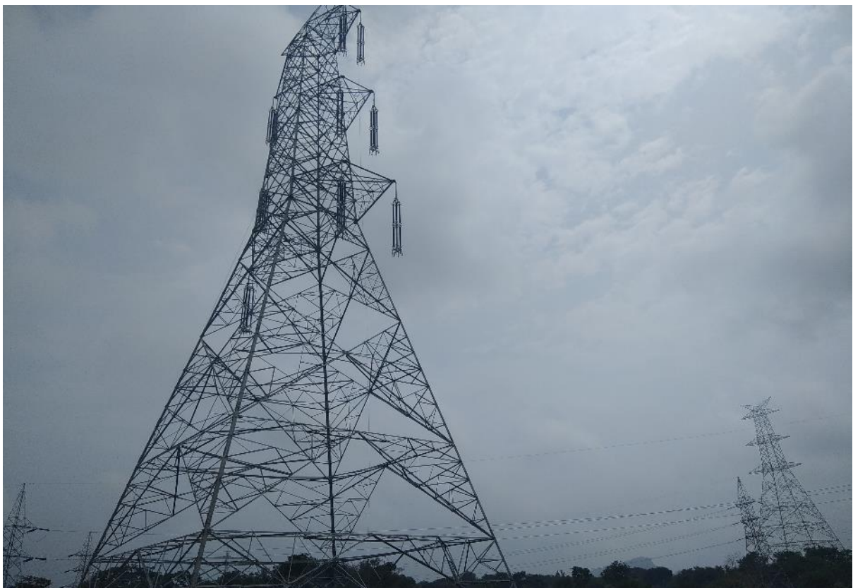
Section 105/0 & 106/0 – Stringing works to start
