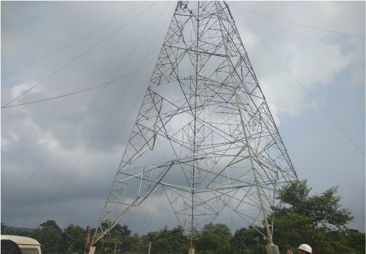
Location 108/3 – Tower erection in progress
