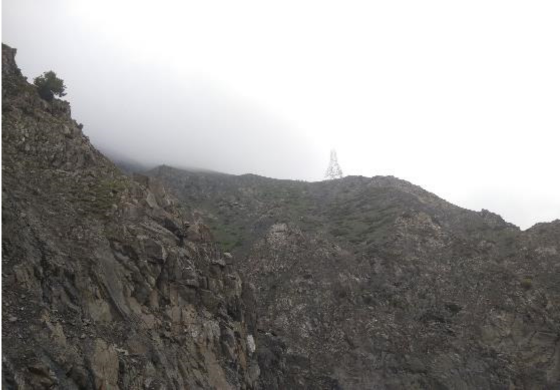
Location 338/1 – Tower Erection in progress
