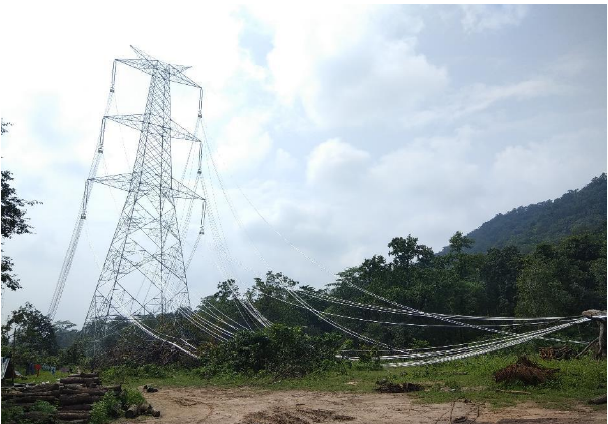
Stretch 115/6 to 116A/0 – Stringing in progress
