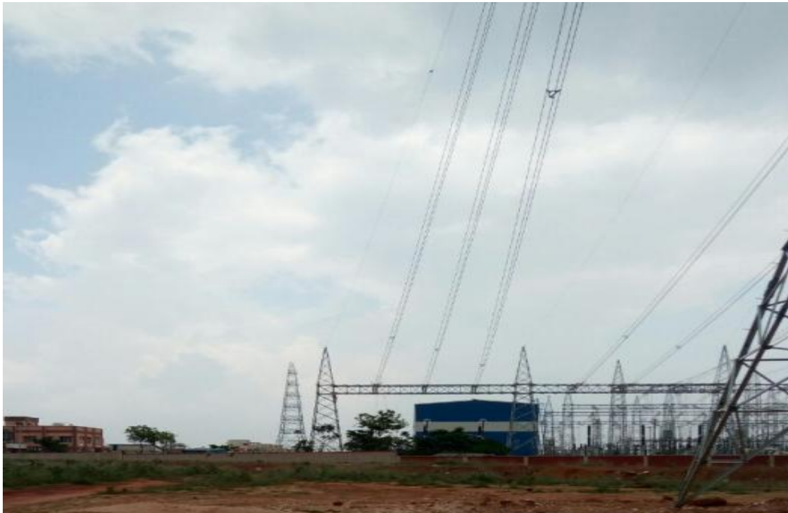
Sundergarh PGCIL substation – Gantry connection complete
