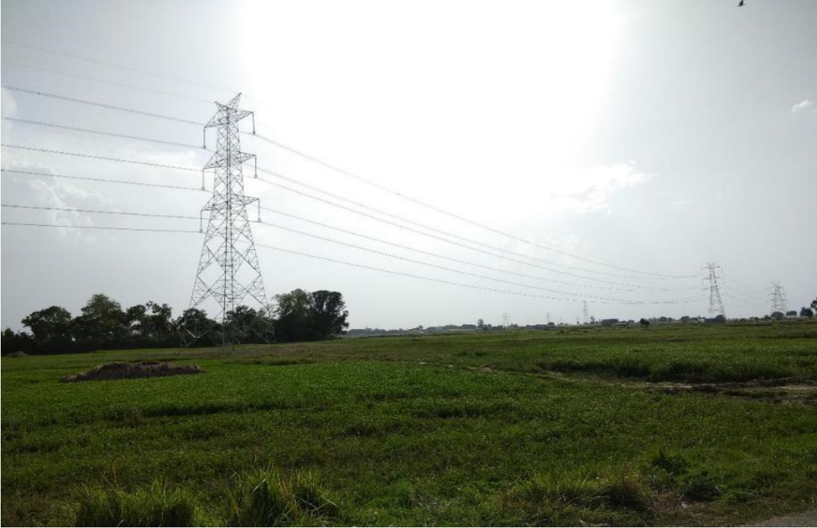
Stretch 20/3 to 30/9 – Stringing complete
