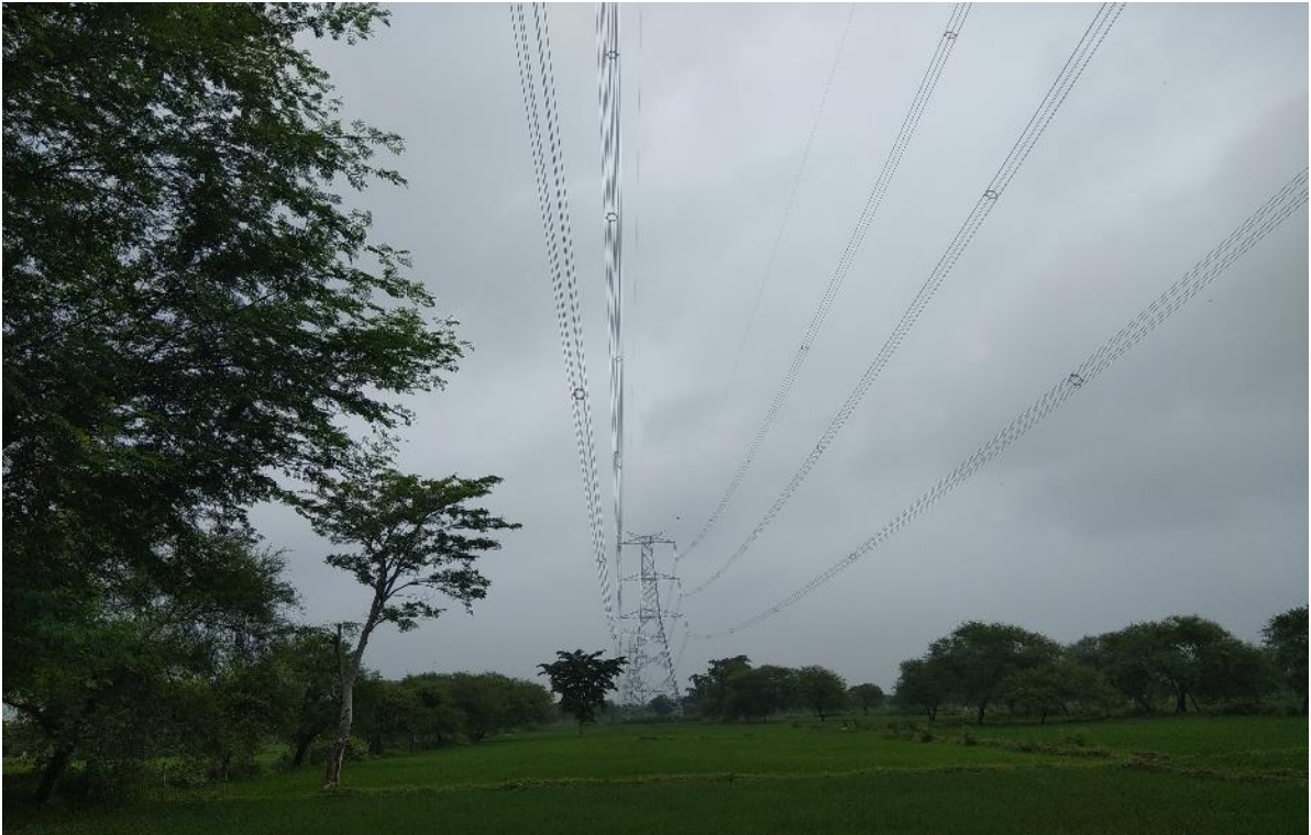
Stretch 1/0 to 4/0 – Stringing complete
