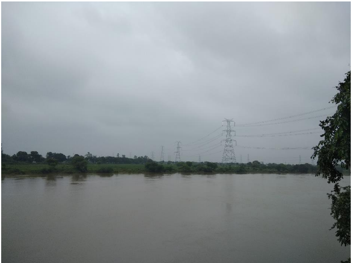
Section 2/3 & 3/0 – river crossing stringing complete
