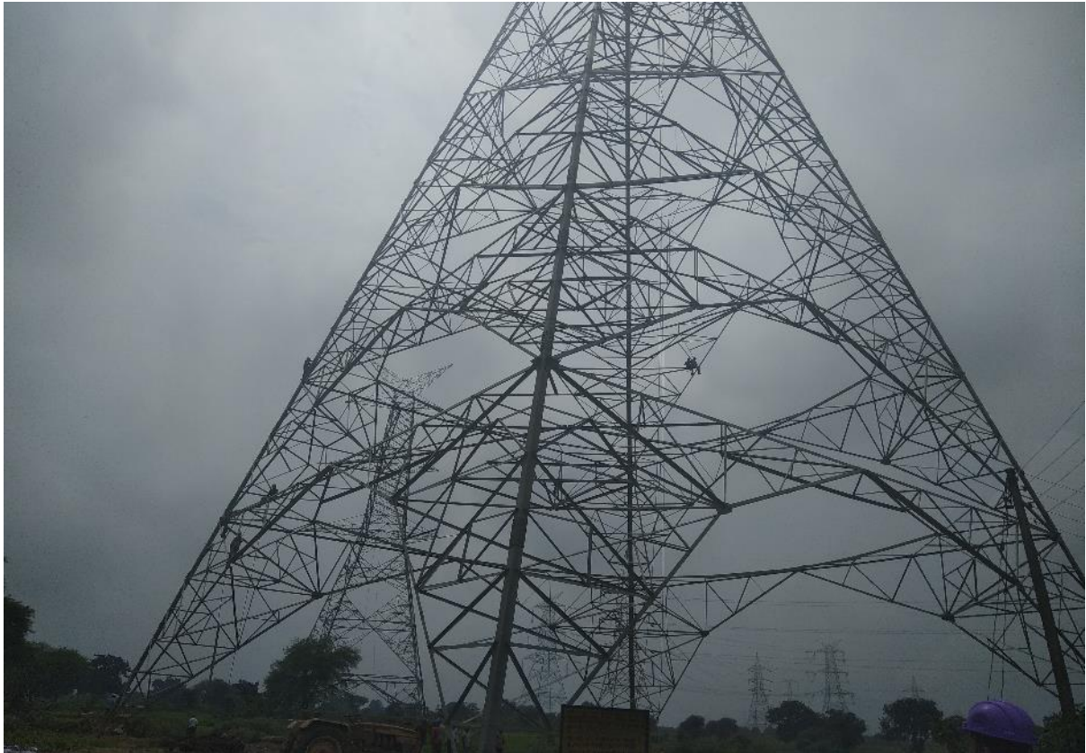
Location 104A/0 – Tower erection in progress
