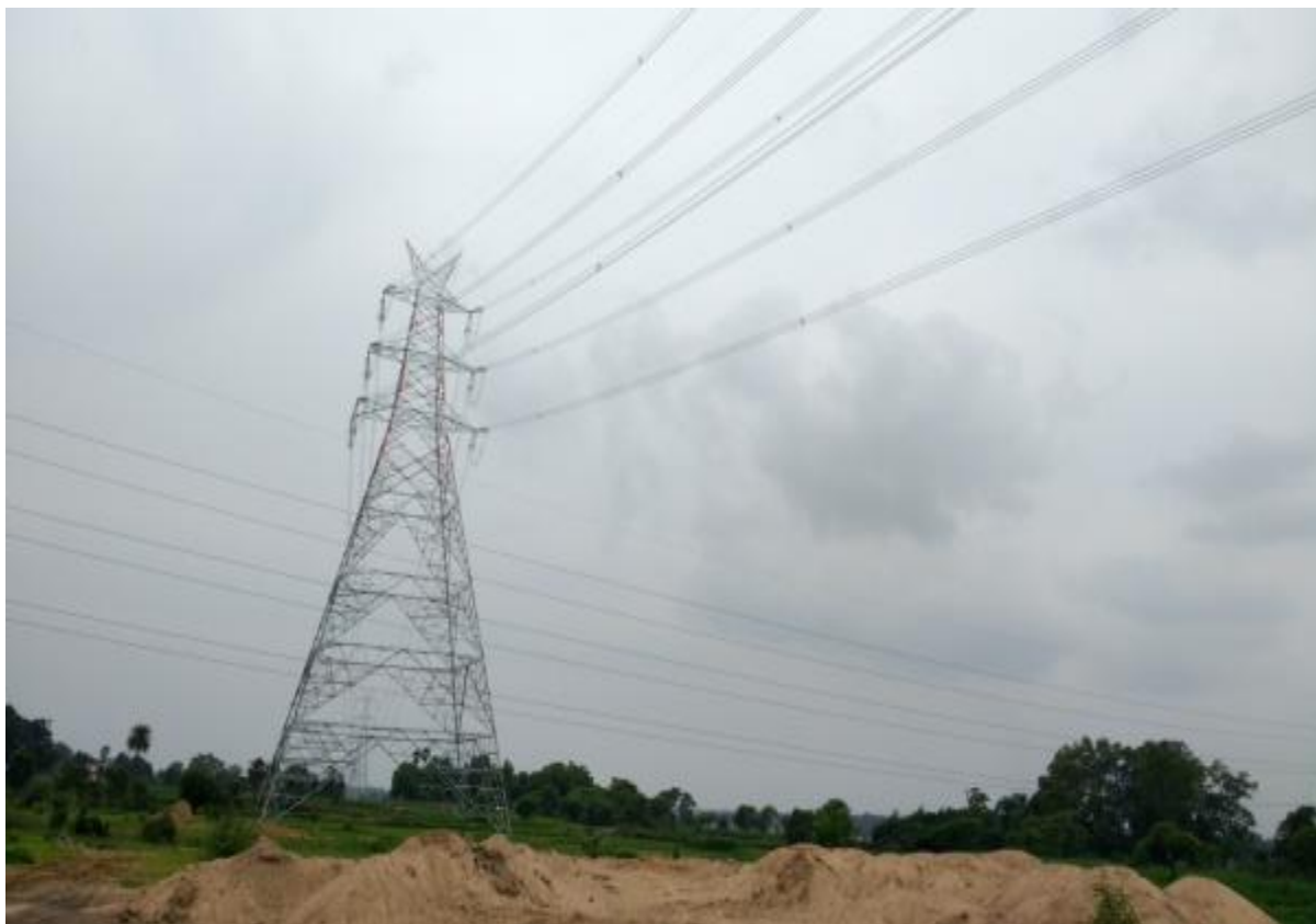
Stretch 32/0 to 33/0 – Stringing complete
