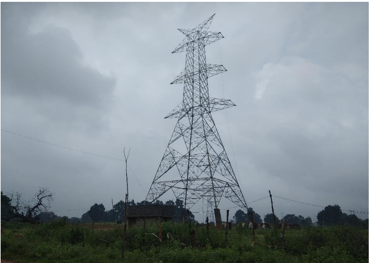
108/4 to 108A/0 – Tower erection complete
