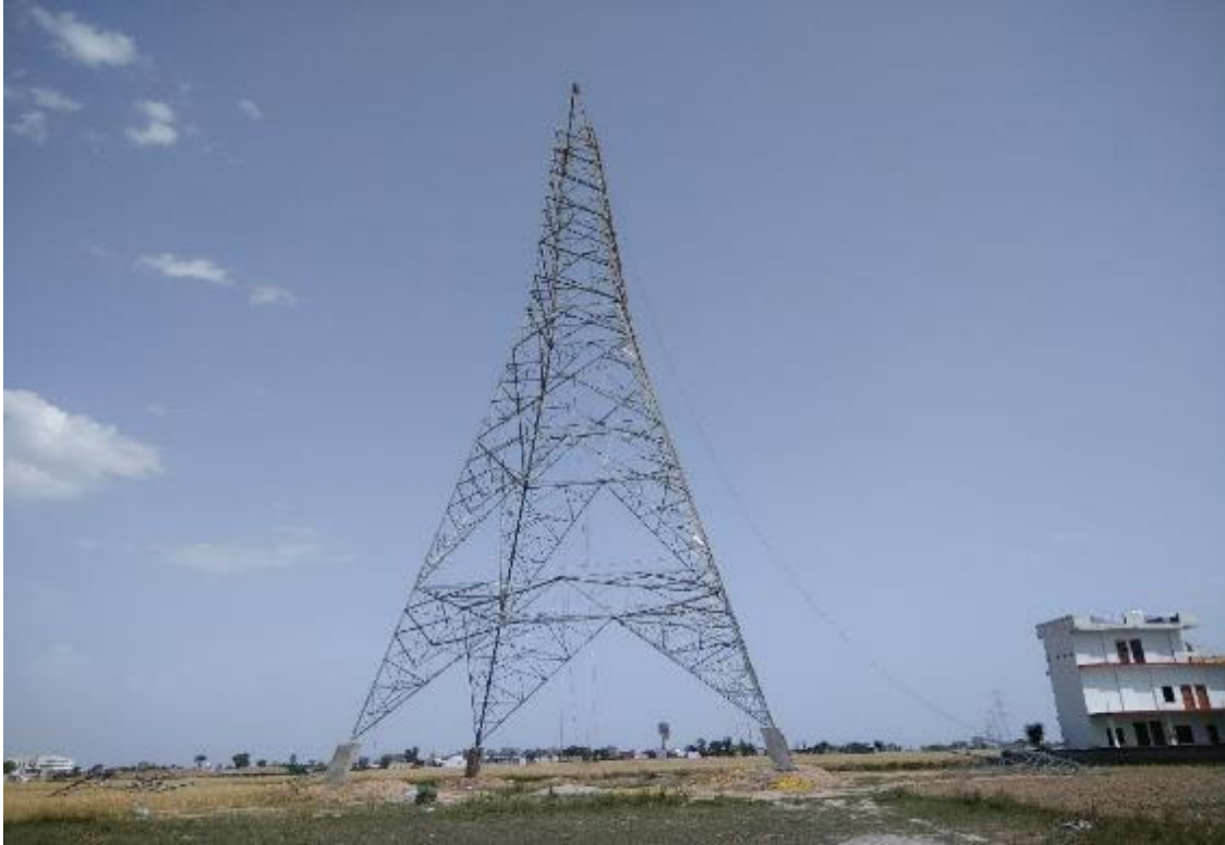
Location 34/0 – Tower erection in progress
